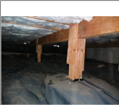
Typical post and beam Construction
