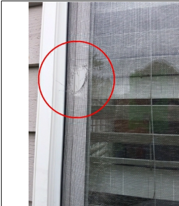
Damaged window screen
