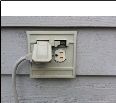
Damaged weather protection cover
