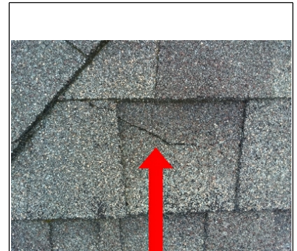
Cracked shingles present
