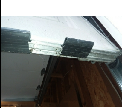
Damaged garage door weather stripping
