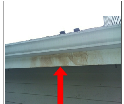
Leaking gutter
