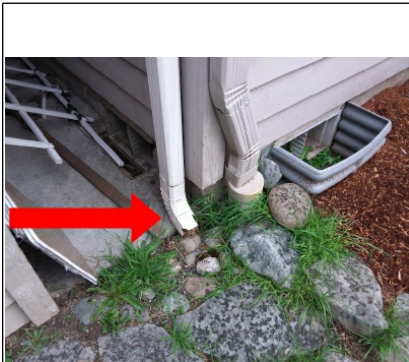
Gutter extension needed
