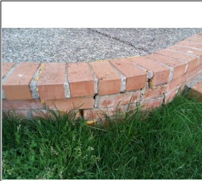
Cracked brick present
