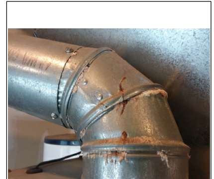
Rust present on furnace vent pipe
