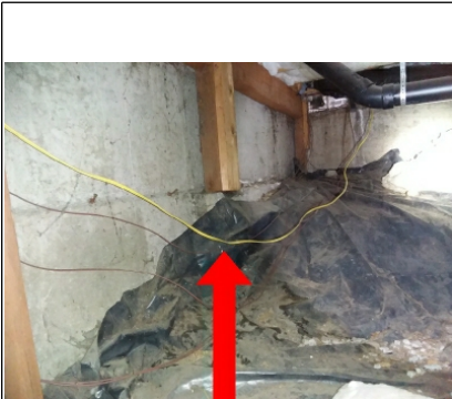
Unsecured electrical wire
