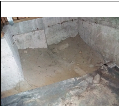
Missing vapor barrier
