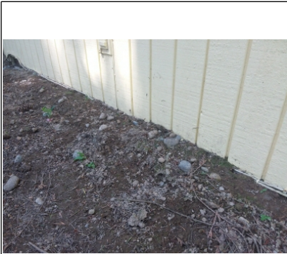
Siding in contact with soil
