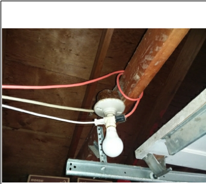
Extension cords to use for permanent wiring
