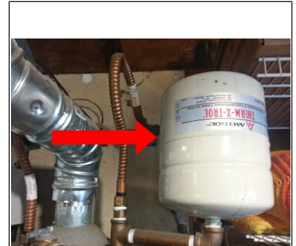
Leaking water heater expansion tank
