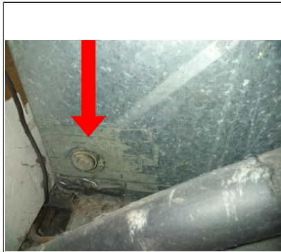
Warm air blowing out of secondary drain hookup
