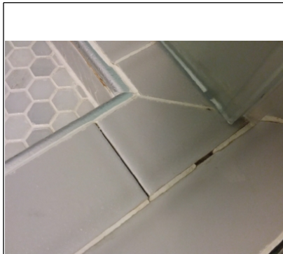
Cracked tile grout present
