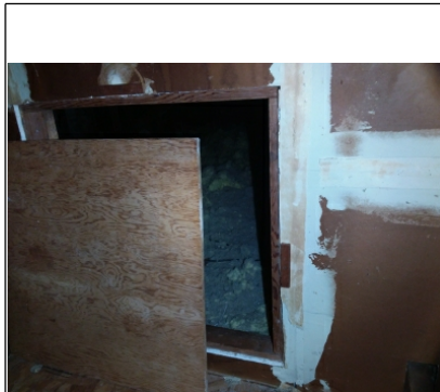
Attic access door is not fire rated
