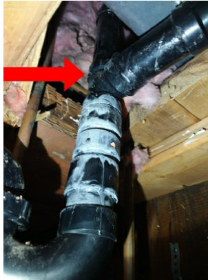
Improperly attached ABS bathtub drain pipe
