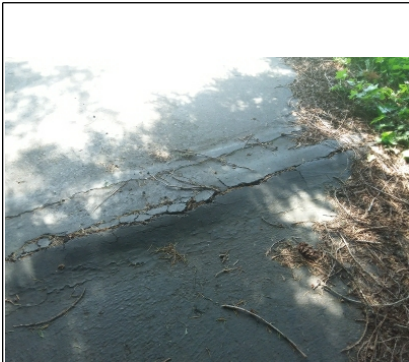
Asphalt driveway has heaved
