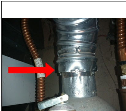
Improper attachment of water heater vent pipe
