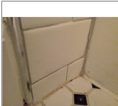
Cracked grout present
