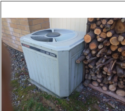
Firewood stacked up against compressor
