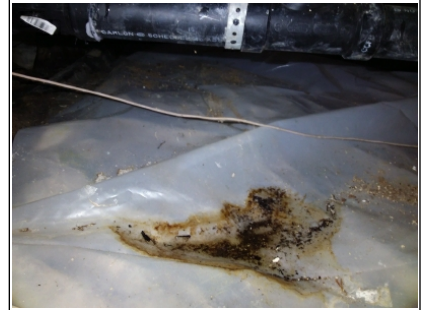
Small puddle of water present under improperly attached drain pipes
