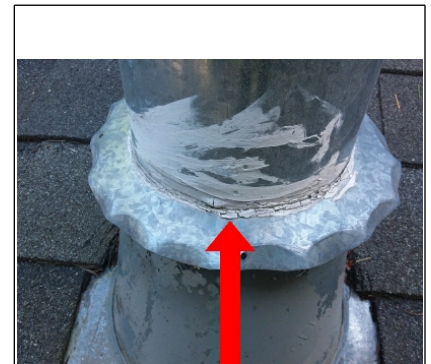
Deteriorating caulking present
