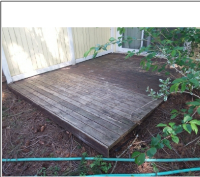
Deck in contact with soil
