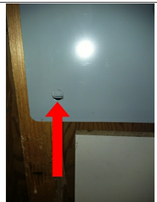
Missing dead front screws
