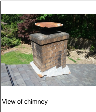
View of deteriorating chimney flashing caulking
