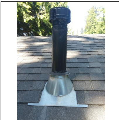
View of gas vent chimney
