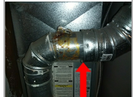
Different types of furnace vent ducting used
