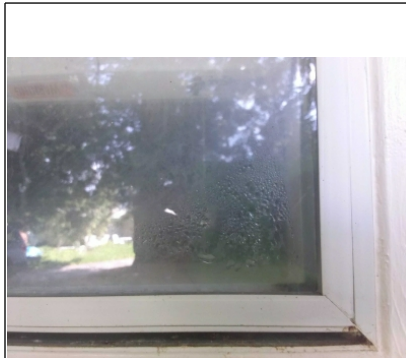
Moisture trapped between window panes
