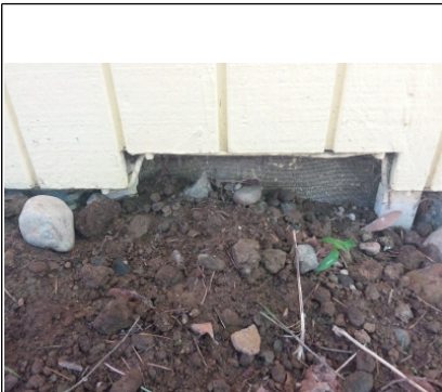
Block crawl space wall vents
