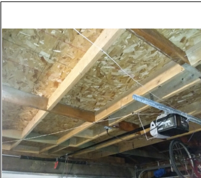
Sagging roof rafters from overhead storage
