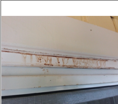
Cracked caulking present above deck sliding glass door
