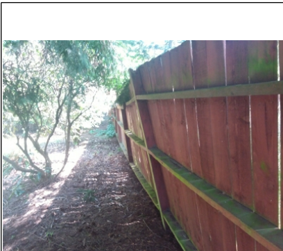
Neighbors wood fence is collapsing
