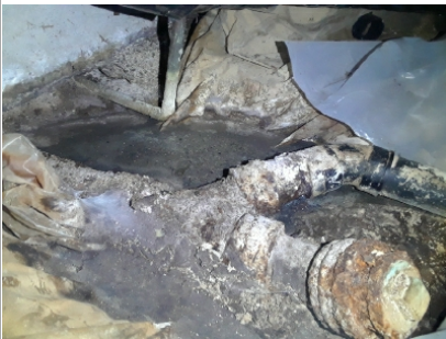
Deteriorating cast iron waste water drain pipe with raw sewage
